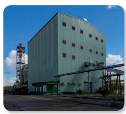
Since 2008, all bark waste along with sewage treatment plant sediments have been burned to produce thermal energy in a large-capacity waste-heat boiler, and the ash generated by waste incineration is cooled and disposed in an environment-friendly manner.
